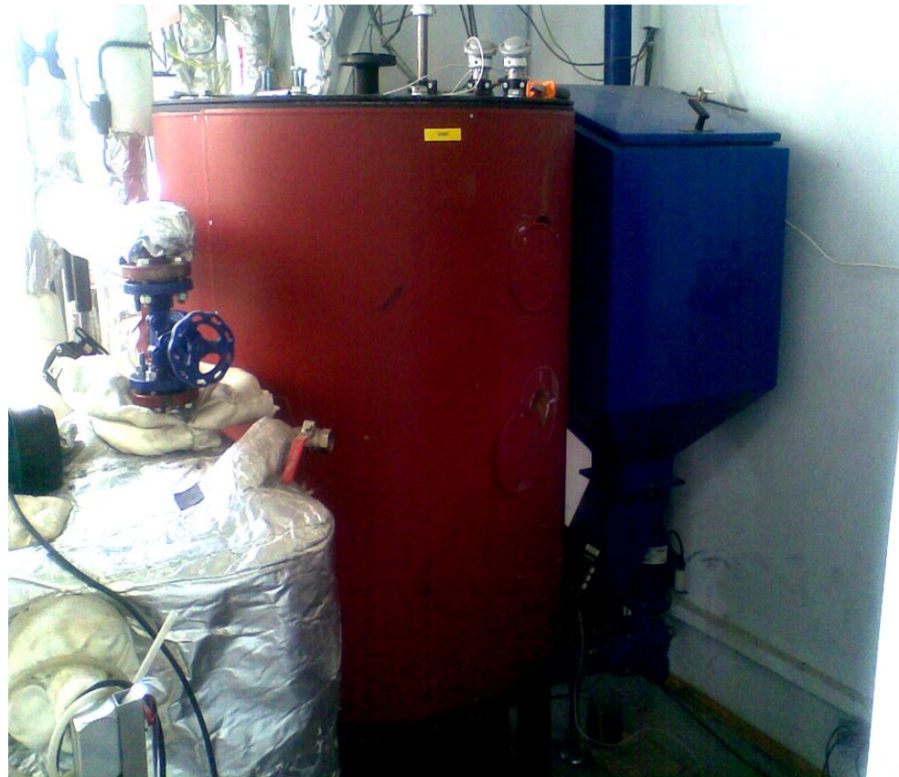
Prototype of multi-fuel boiler with a solid fuel reservoir (biomass-pellets).
