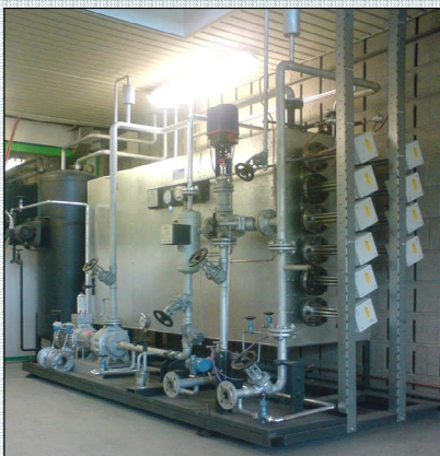
Heat source: Thermal oil boiler 250kW, Maxxtec
